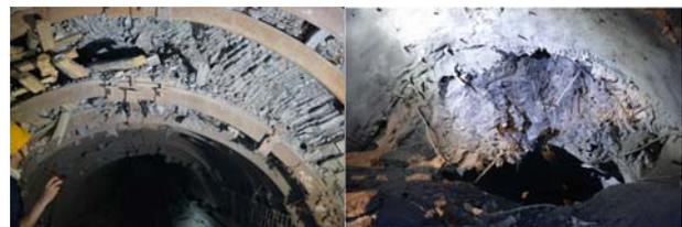
Fig. 16 Roadway damage under the original support scheme
