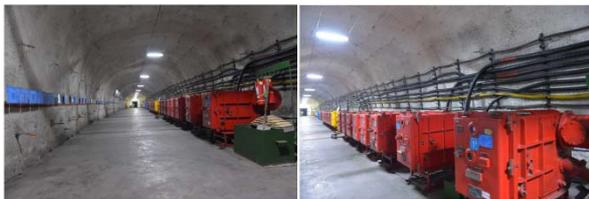
**Fig. 19** Substation roadway with new prestressed anchoring and reinforcement
