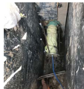
Fig.8 Installation of displacement meter
